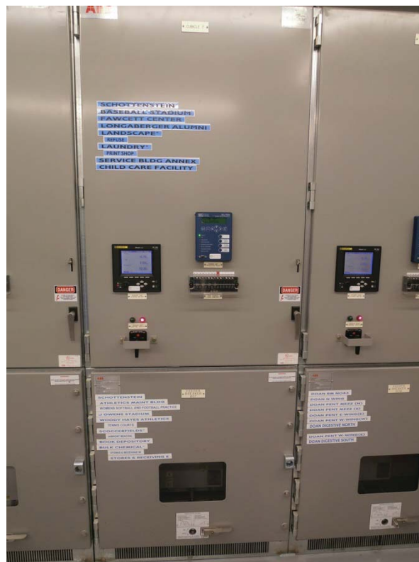
Street Feeder Switchgear Panel—front view
