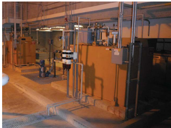
Smith Standby DG Day Tanks
