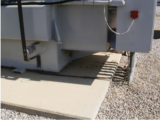
Main Transformer Grounding
