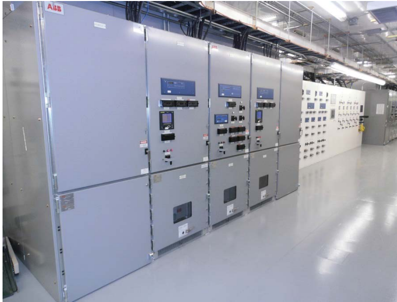
Main-Tie-Main at WCS
