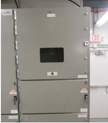
Examples of Potential Transformer Installations PT Compartment in Switchgear (left) Structure mounted PT (right)
