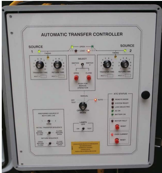
Standard Primary Switch Transfer Control
