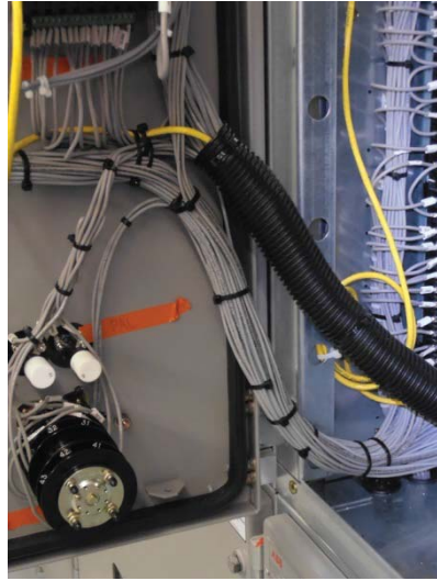
Figures showing good wiring practices Note wire bundle crossing hinge area (left) and cable training area and labeling (right)
