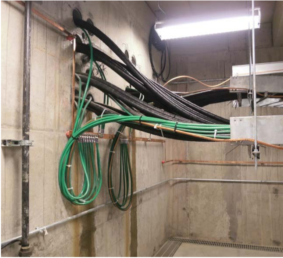
Distribution System Ground Cable Grounding
