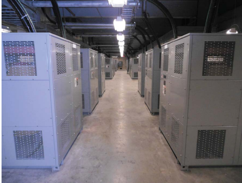
600-Ampere 15 kV Class Reactors
