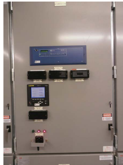
Main Feeder Breaker
