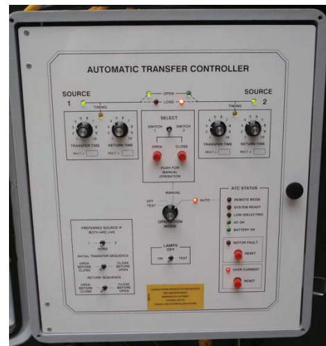
Standard Transfer Controller Box
