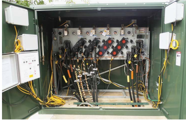
6-way Primary Switch Enclosure Showing 4 RFI Trip Units and Transfer Box
