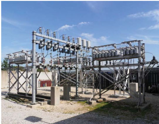
OSU Outside CAP Bank Design (3 banks)
