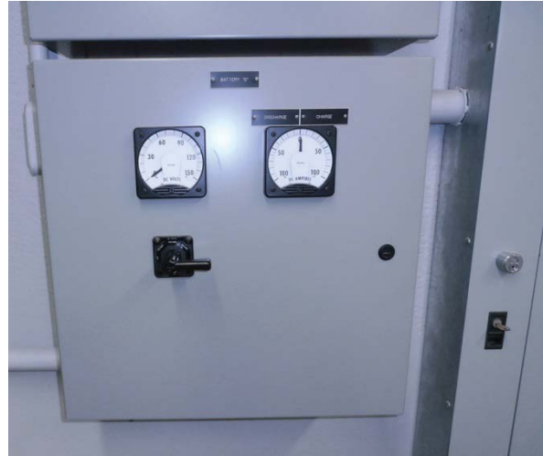
DC Battery Meter Compartment
