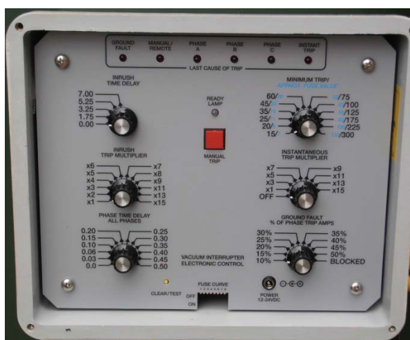
Current Multifunction Trip Module
