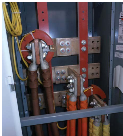
Figures showing bad wiring practices Note CTs mounted on bus (left) and use of mechanical connectors (right)
