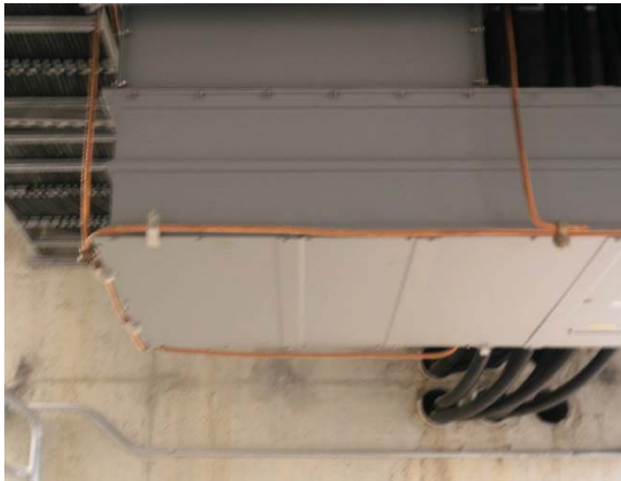
Non Segregated Bus Duct Grounding
