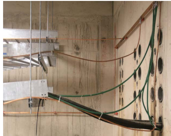
MV Tray and Cable Grounding
