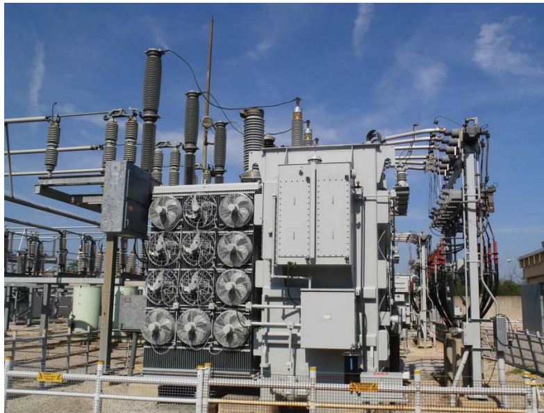
Side View of OSU Sub Transformer 138 kV enters from the left, 38 kV on pilaster right
