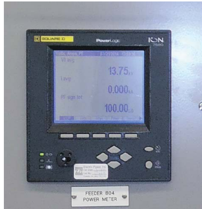
3-Phase Meter on Switchgear
