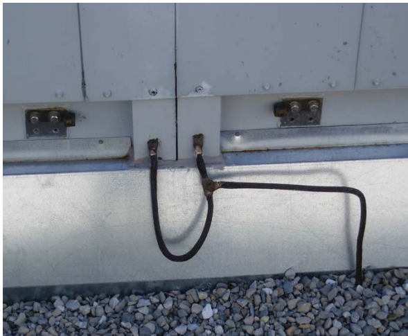
WCS Equipment Enclosure Grounding
