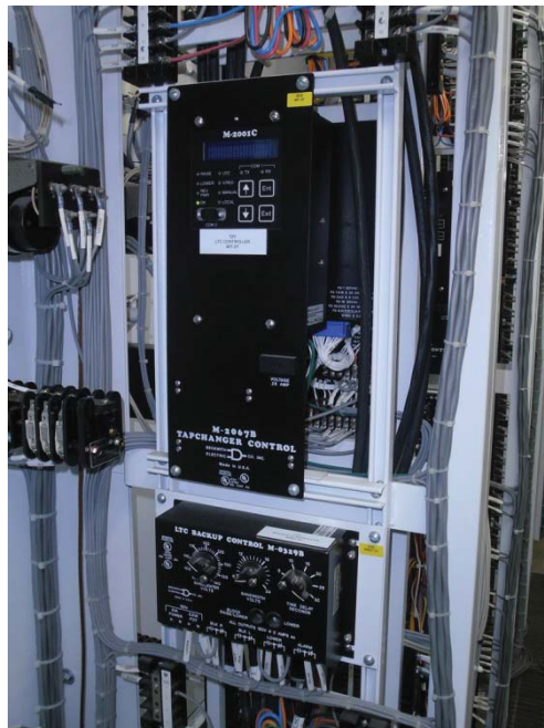
DeltaVar Controller and Front Panel Main Controller (top) Backup Controller (bottom)
