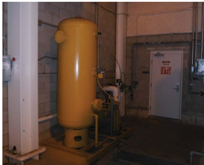
Smith Standby DG Starting Air Package
