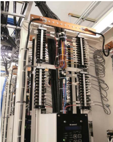
Main Control Panel upper ground buss
