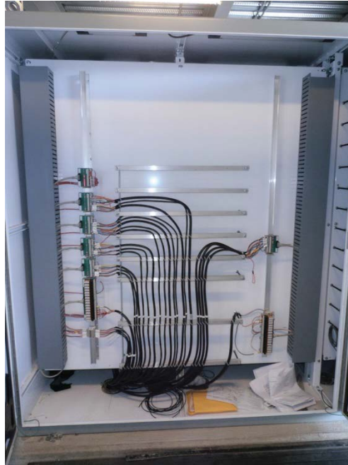
Typical Logic Panel Termination Compartment
