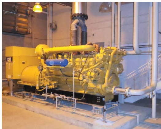
Smith Standby Diesel Generator
