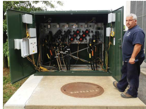
Primary Switch Terminations
