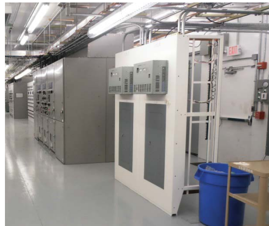
Standalone UPS at McCracken (left) and Paired Units at WCS (right)
