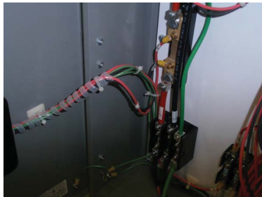
Figure showing a bad wiring practice Door wiring traverses hinge area and places loading directly on terminations in cabinet
