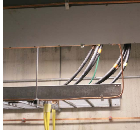
Electrical Tray Grounding
