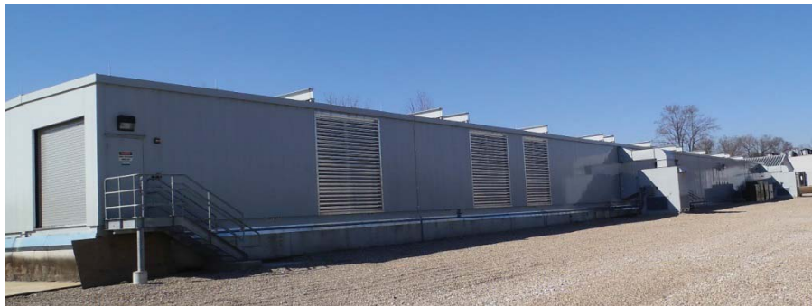
West Campus Substation Equipment Enclosure
