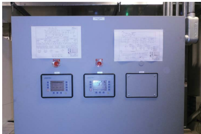
EasyGen DG HMI on SCCC DG Generator Control Panels
