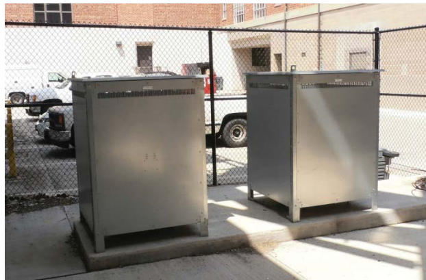
SCCP Standby DG Grounding Banks
