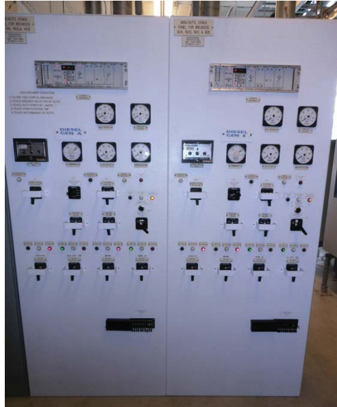
Smith Sub DG Paralleling/Sync Panel
