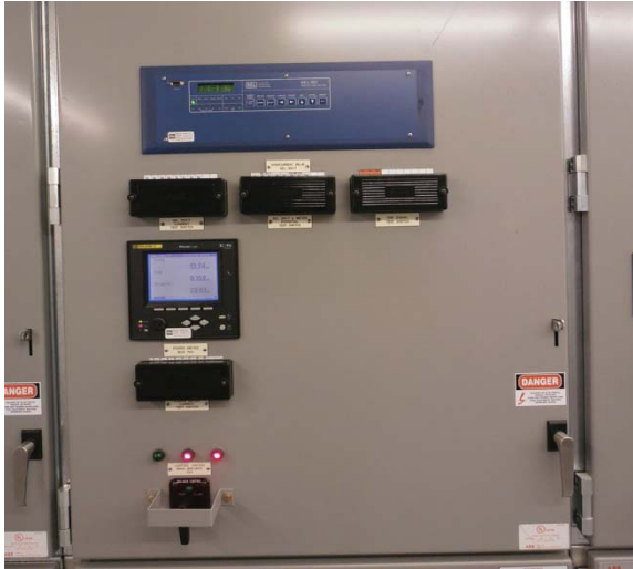
Good label Labeling minimal and task oriented
