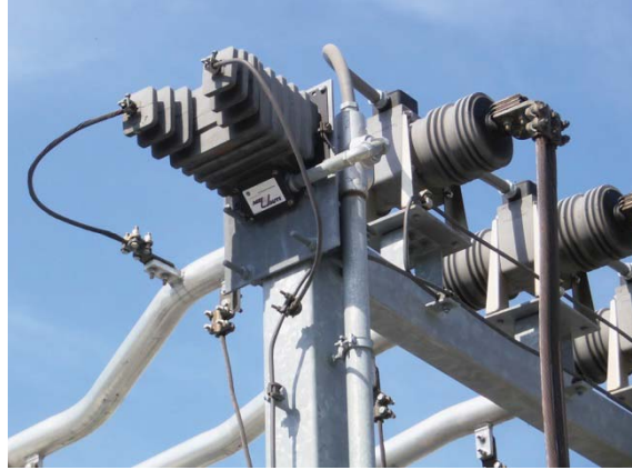
Examples of Potential Transformer Installations PT Compartment in Switchgear (left) Structure mounted PT (right)
