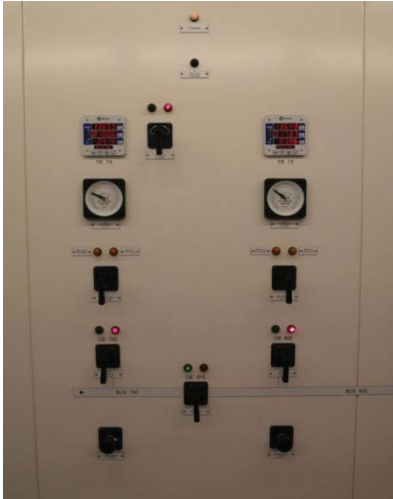
Main Transformer Control Board
