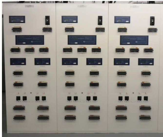
WCS Transformer Protection Panels
