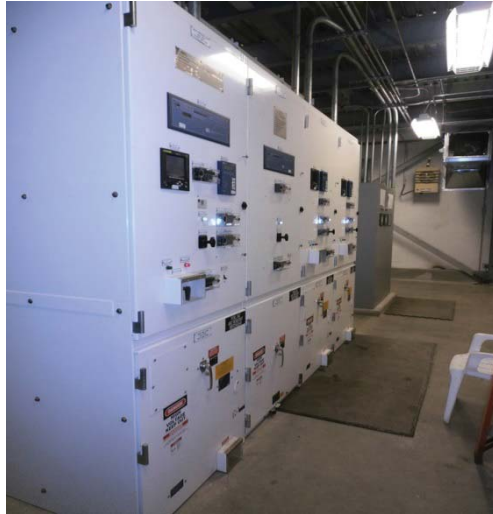
SCCCP Paralleling Gear SCCCP Paralleling Gear (left); Woodward EasyGen HMI (right)
