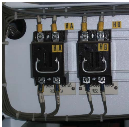
Typical Switchgear ganged DC fuse Application
