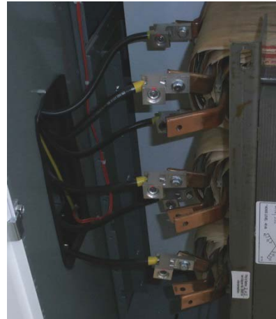
Figures showing bad wiring practices Note CTs mounted on bus (left) and use of mechanical connectors (right)
