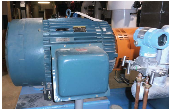
Oversized Motor Terminal Box
