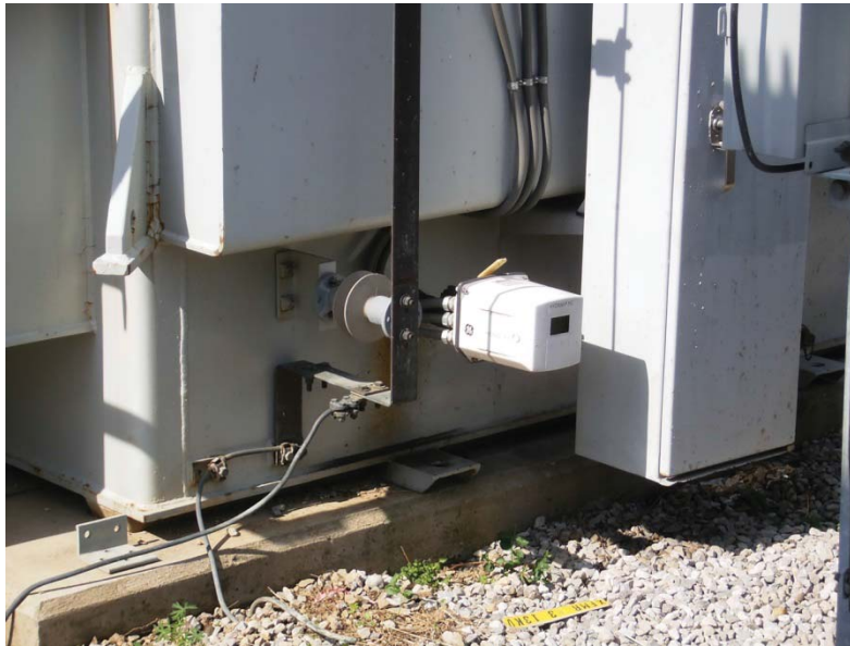
Hydran Installation
